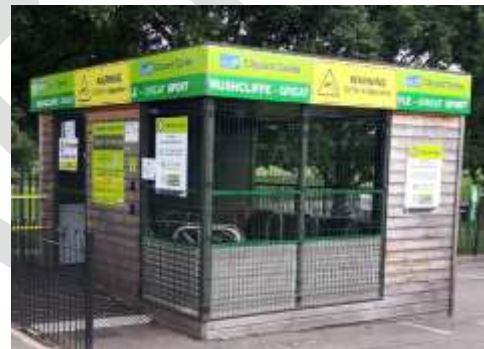
Secure Cycle Hub in Bridgford Rd Car Park
